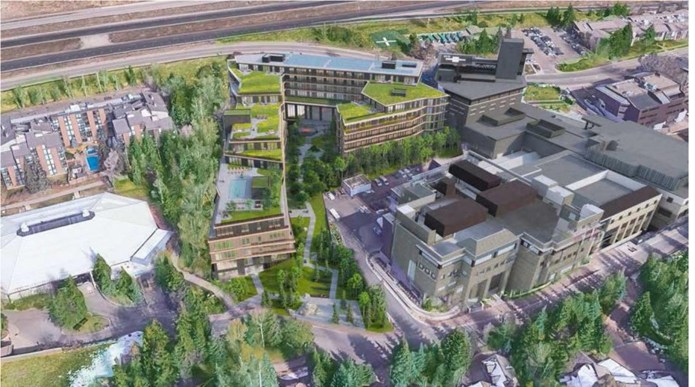
Proposed redevelopment of Evergreen Lodge (center) located west of Vail Health campus on West Meadow Drive.
