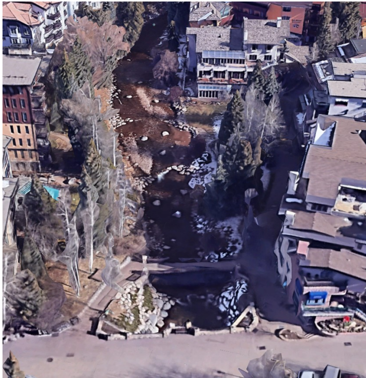
Aerial view of Gore Creek and Promenade.
