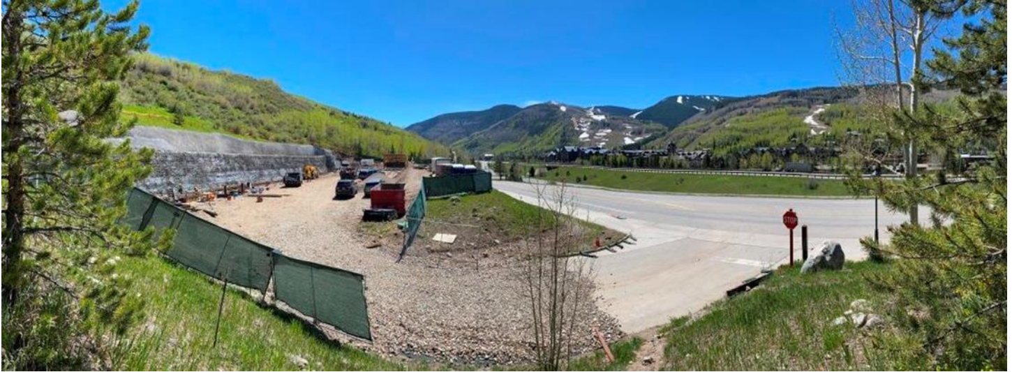
Residences at Main Vail under construction.
