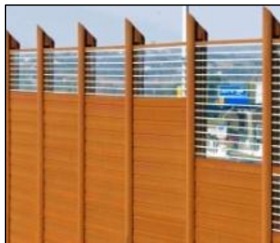
Above: Transparent acrylic glass sound wall attached to concrete crash barrier on the Autobahn between Innsbruck, Austria and Munich, Germany
