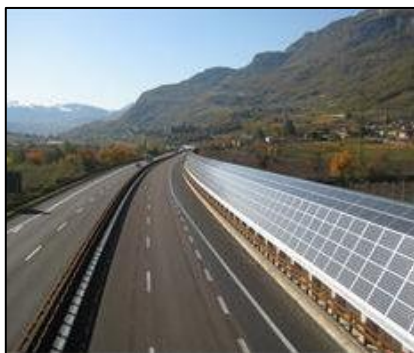
Above: Transparent acrylic glass sound wall attached to concrete crash barrier on the Autobahn between Innsbruck, Austria and Munich, Germany
