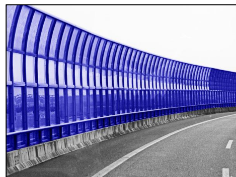
Above: Transparent acrylic glass sound wall attached to concrete crash barrier on the Autobahn between Innsbruck, Austria and Munich, Germany
