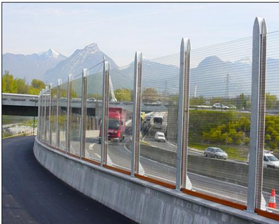
Above: Transparent acrylic glass sound wall attached to concrete crash barrier on the Autobahn between Innsbruck, Austria and Munich, Germany
