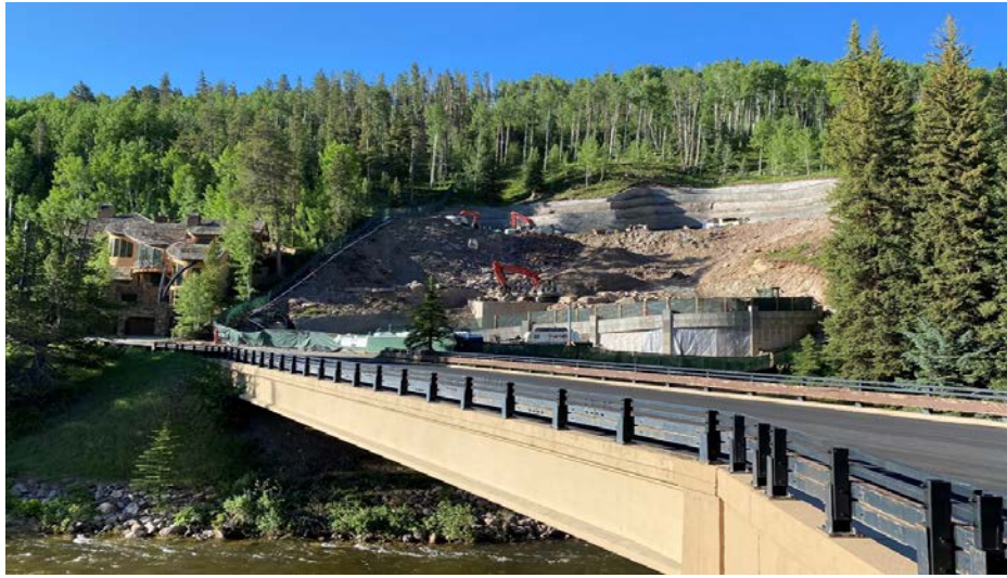
West Forest Road Construction - How and why did this happen?
