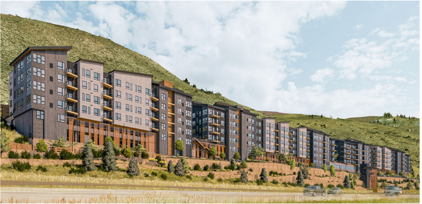
Architect's rendering of West Middle Creek from I-70, opposite the Town Center of Vail Village and Lionshead. Indebted by bond funding, currently under construction.
